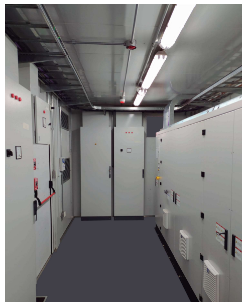
Detalle interior del Shelter
